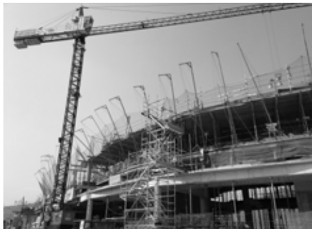
DATA CENTER BANCOMER
