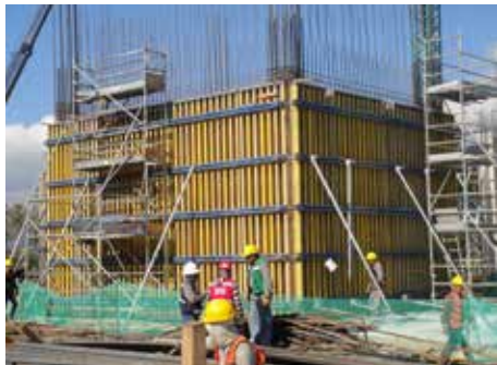
DATA CENTER BANCOMER
